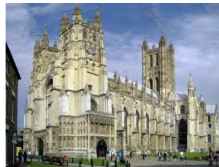
Canterbury Cathedral (built 1070)
